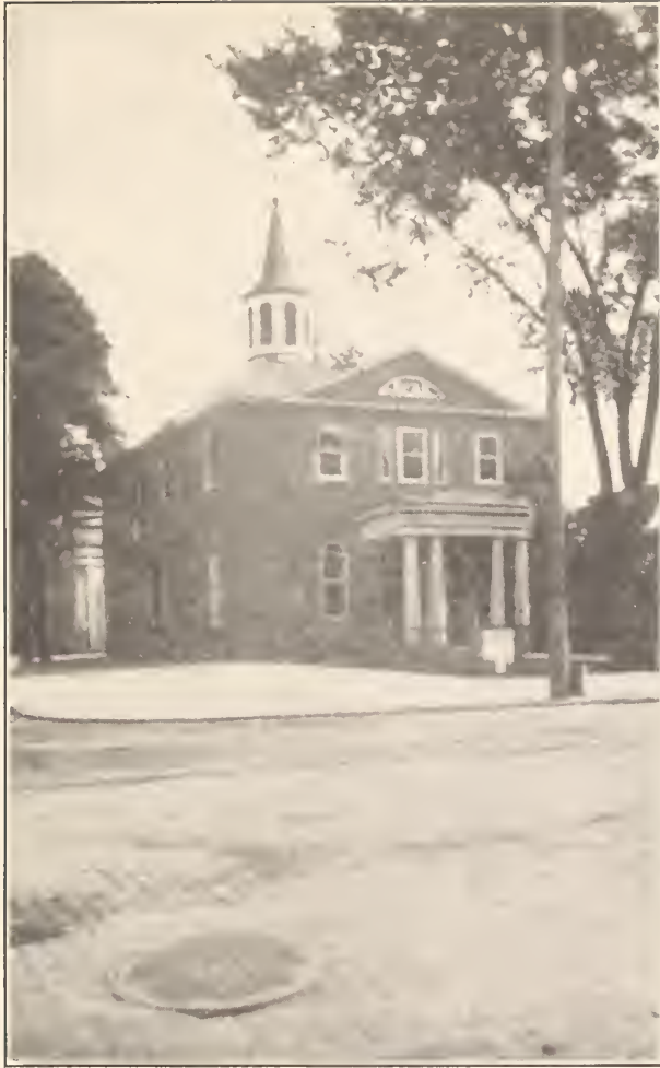
COURT HOUSE, SALEM
